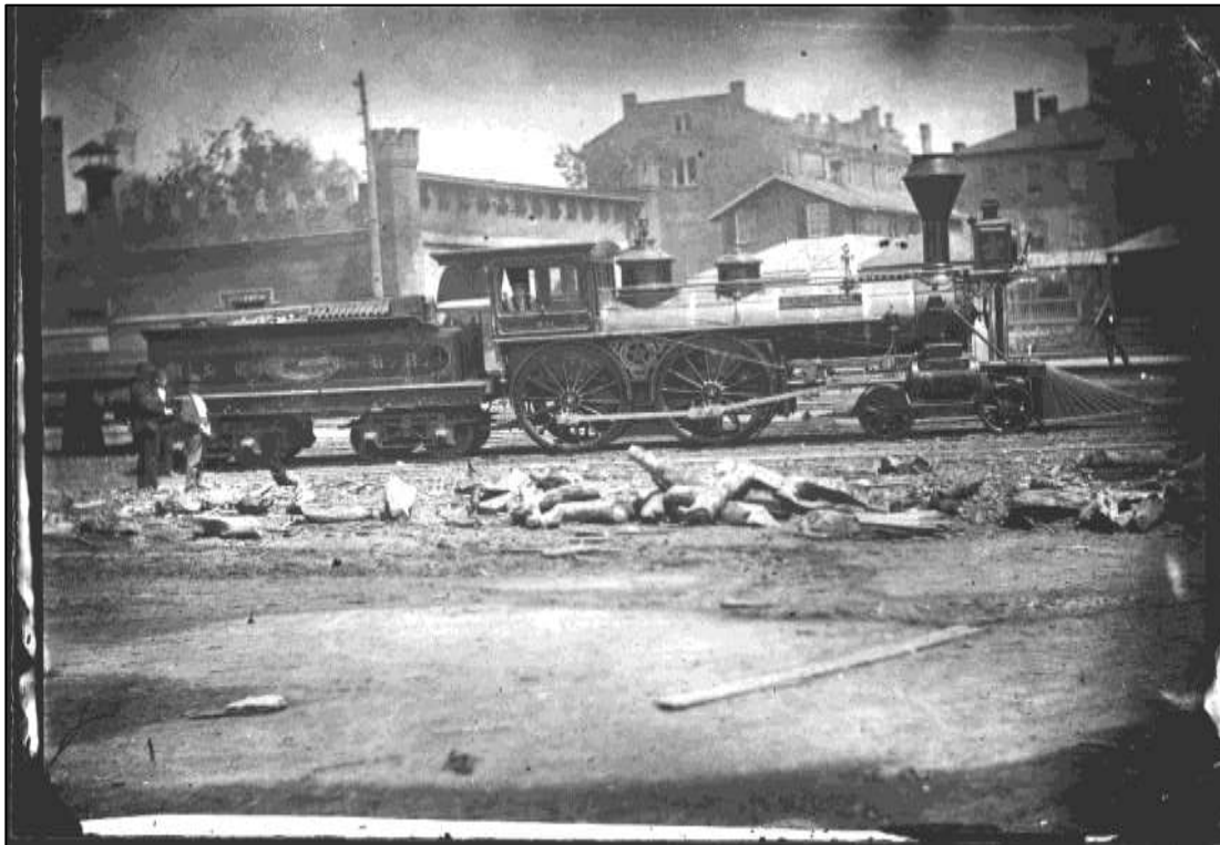
A locomotive stands in front of the Louisville & Nashville railroad depot on Church Street in Nashville, ca. 1870. The depot is the building with turrets just behind the train. The taller building to the rear is thought to be the Nashville Female Academy. (Library Photo Collection, Tenn. State Library & Archives.)
